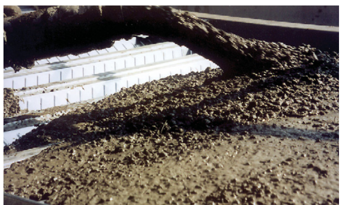
Concrete time savings by using Kingspan MD 60 metal deck and Dramix® reinforced concrete.
